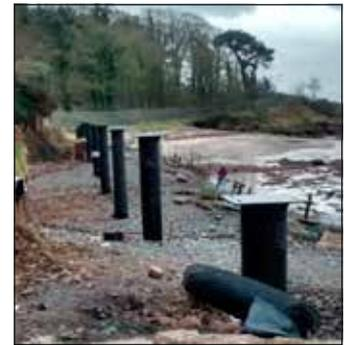
The photograph shows the columns on which the walkway will be elevated, above the reach of the highest tides. Though not quite in the Gobbins Path league, it should provide a dramatic new section for walkers, joggers and cyclists.
